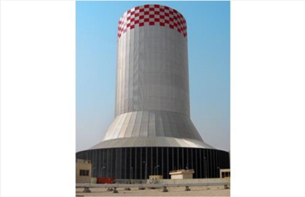
(Air Cooling Condenser) ACC -2
